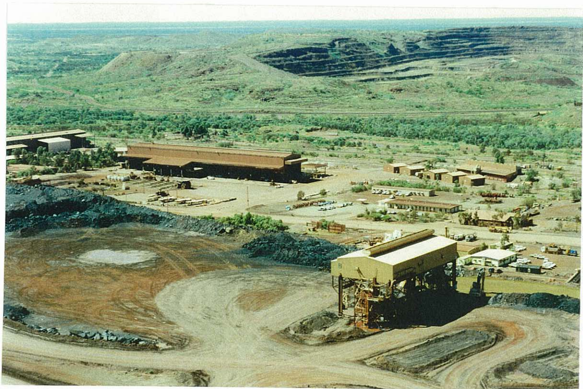
A view of the workshops and the high grade crushing plant No 2. This plant was installed in 1971 and is where iron ore boulders of up to 1.5m in diameter are reduced down to 200mm or less, before going via conveyor belt to a secondary crusher. There the ore is crushed to 100 mm or smaller, and then transported to train loadout stockpiles.
