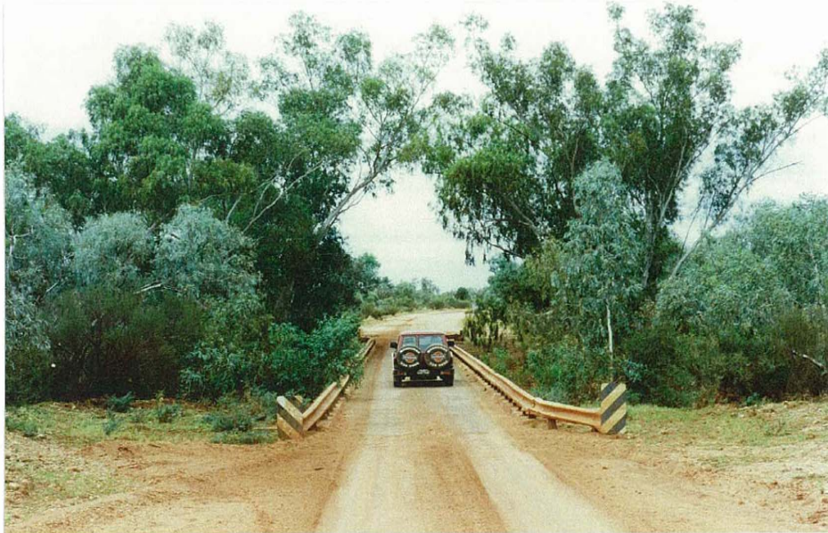
The bridge as seen from the road.
