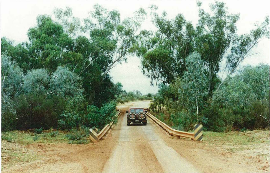
The bridge as seen from the road.
