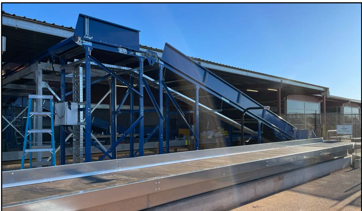
Baggage Carousel Installation Process
